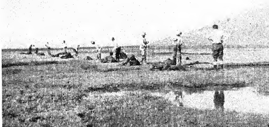
Figure 36. Laborers excavating a drain ditch across a salt marsh
